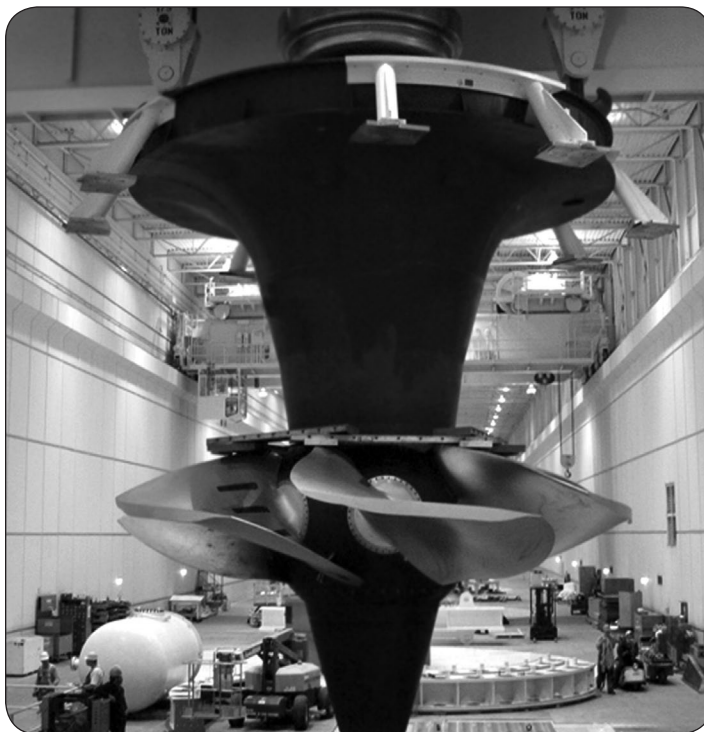
This fish-friendly turbine has openings large enough for fish to pass through.
