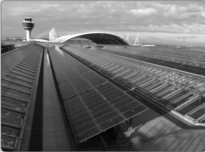
Image courtesy of BP Solar
