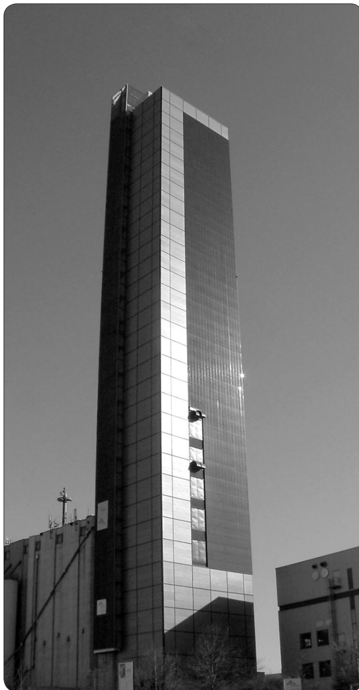
The Schapfen Mill Tower is a flour mill in Germany. The southern facade is faced with 1,300 thin-film solar modules.
