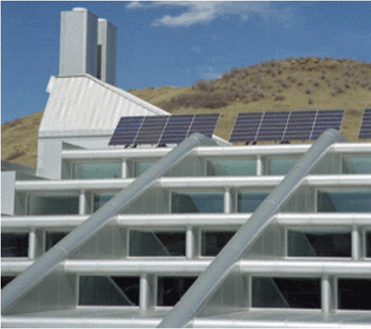
Clerestory windows provide daylighting for workers in this building.
