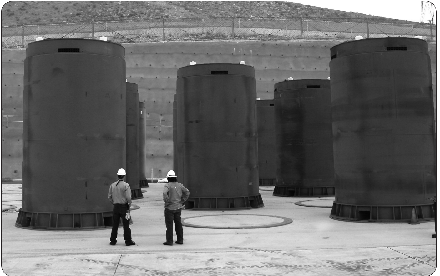
Used nuclear fuel is often stored in large fuel casks.
