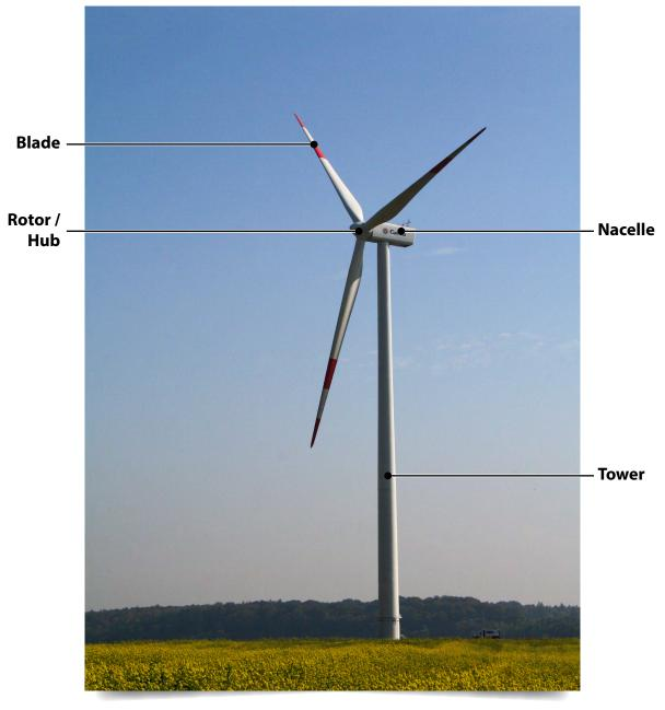
Wind turns the turbine blades, which spin magnets and wires inside the nacelle to generate electricity.
