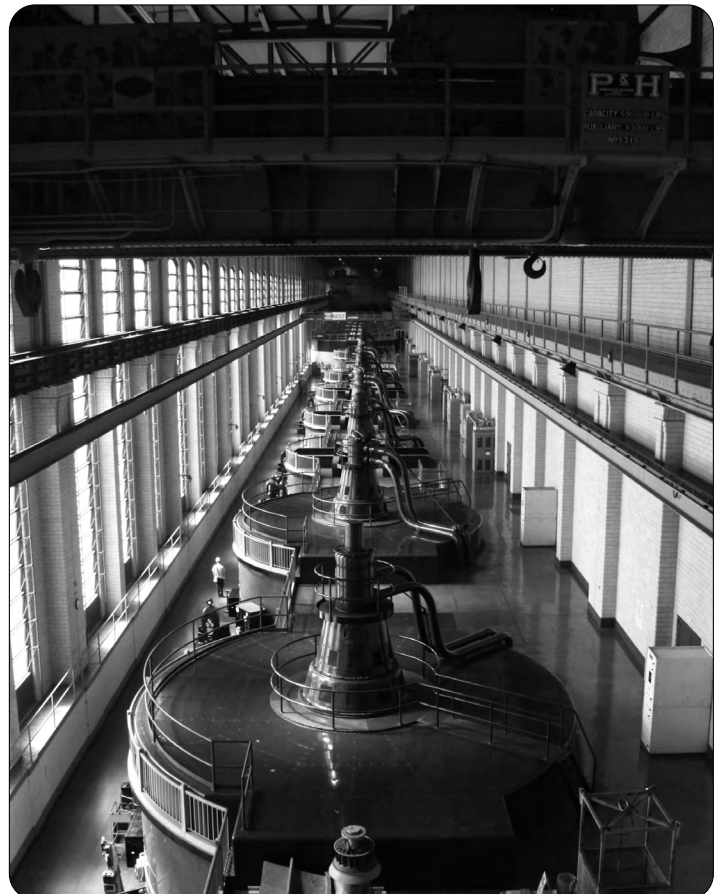
Photo of Safe Harbor Water Power Corporation on the Lower Susquehanna River in Pennsylvania.
